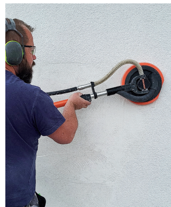
Grinding large surfaces very quickly
