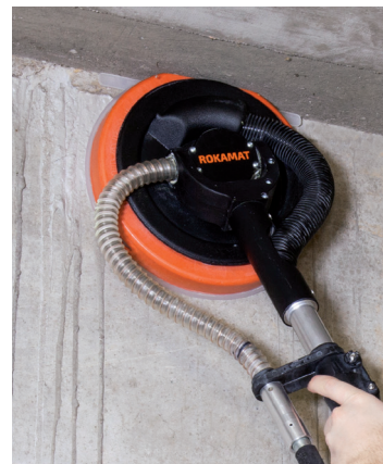
Grinding concrete burrs
